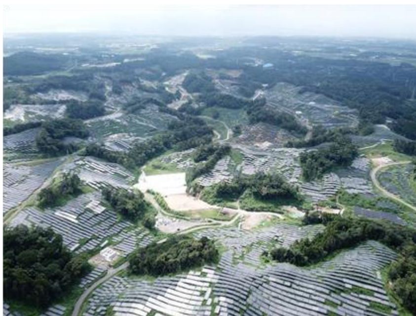
Kanoya Osaki Solar Hills Solar Power Plant
